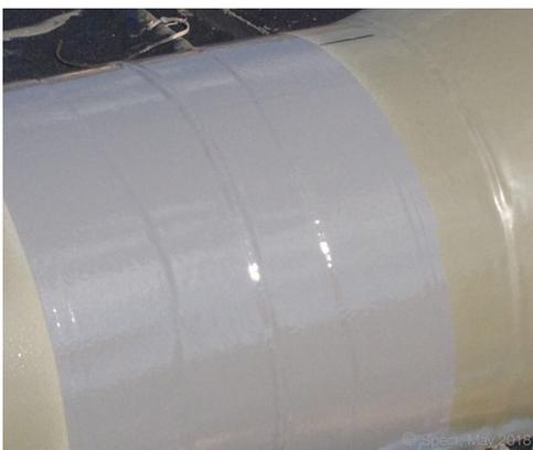
Polyclad 777 weld joint sprayed with MixCoat System
