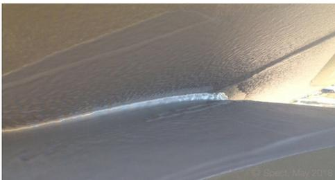
Sulzer Mixpac Dual Flex Line works even for pointed angle tee pieces (Polyclad 777 full seal over weld)
